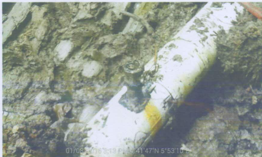
POINT DURING EXCAVATION: fig 2
